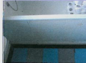
◀ Asbestos cement bath panels
